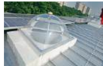
Rotating mirrors installed at the end of a light pipe
