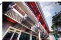
Light travels through duct via multiple reflection
