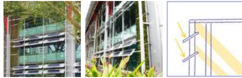
Figure shows the impact of shading on consumption of energy for cooling purpose
