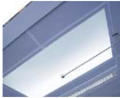
Openings in the duct and false ceiling allow daylight to exit and illuminate the interior space.
