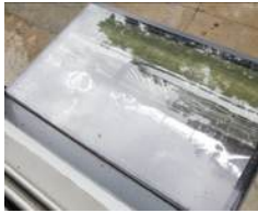
Top view of the mirror duct's external collector.
